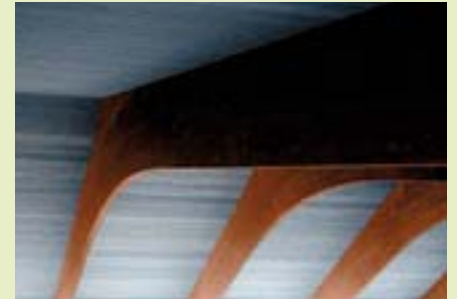
GLT™ Mono tongue/groove as a visible supporting and bracing ceiling.
